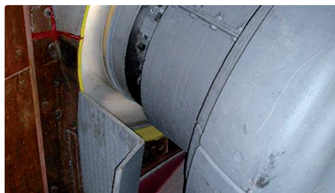
Flexible seal between housing and roller
