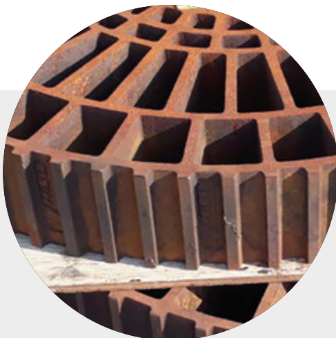
BEFORE THE REPAIR SERVICE
